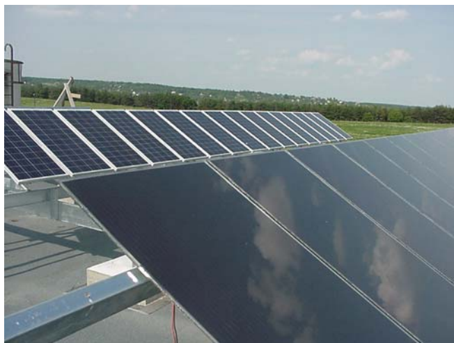
Figure 1. The two PV module types of system (DS40 in the front, ASE-100 in the background)
