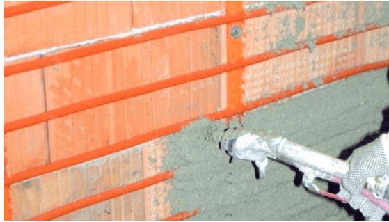
Figure 3. Plastering with mortar sprayer machine
